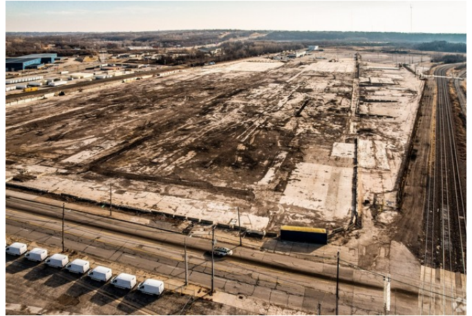
Former GM Leeds site following demolition
