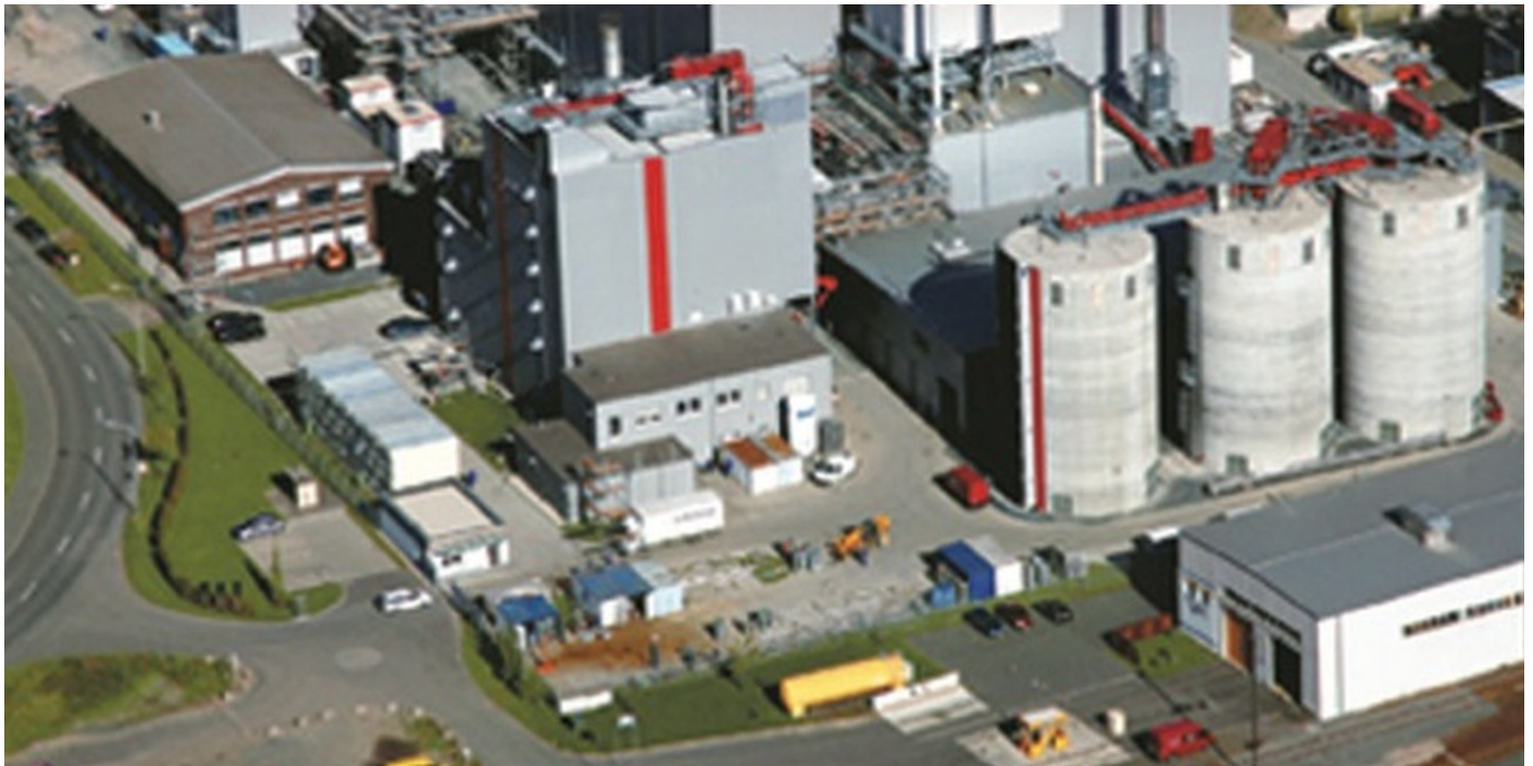
CHOREN facility in Freiberg, Germany
