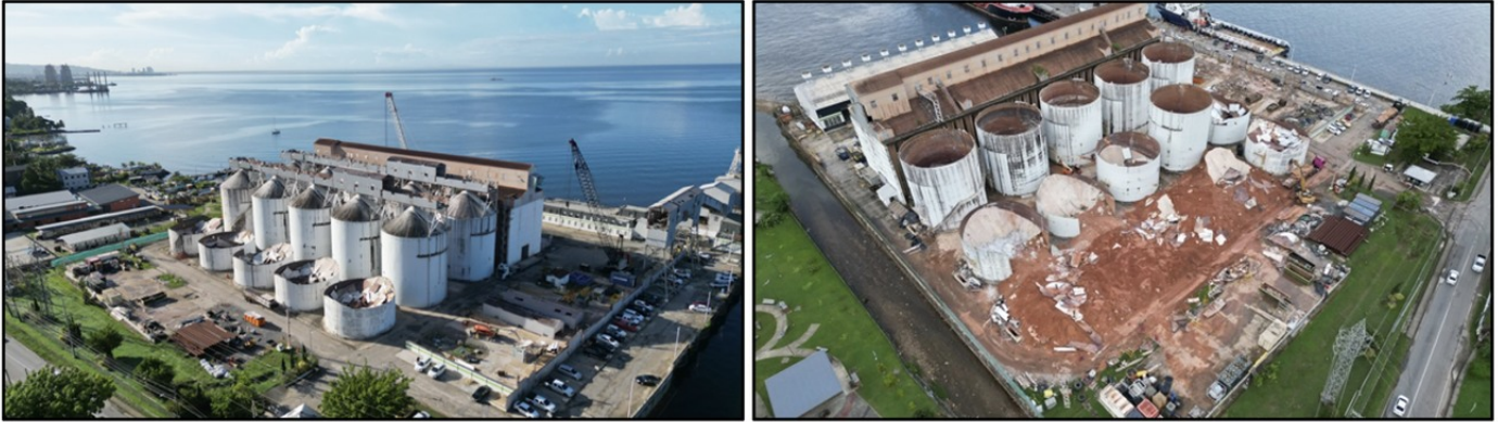
Tembladora facility before and during dismantlement
