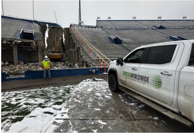
Winter demolition at KU Jayhawk Stadium
