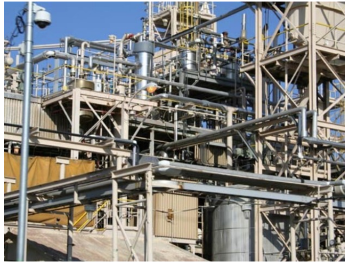
Big River Zinc process structures, Sauget, Illinois
